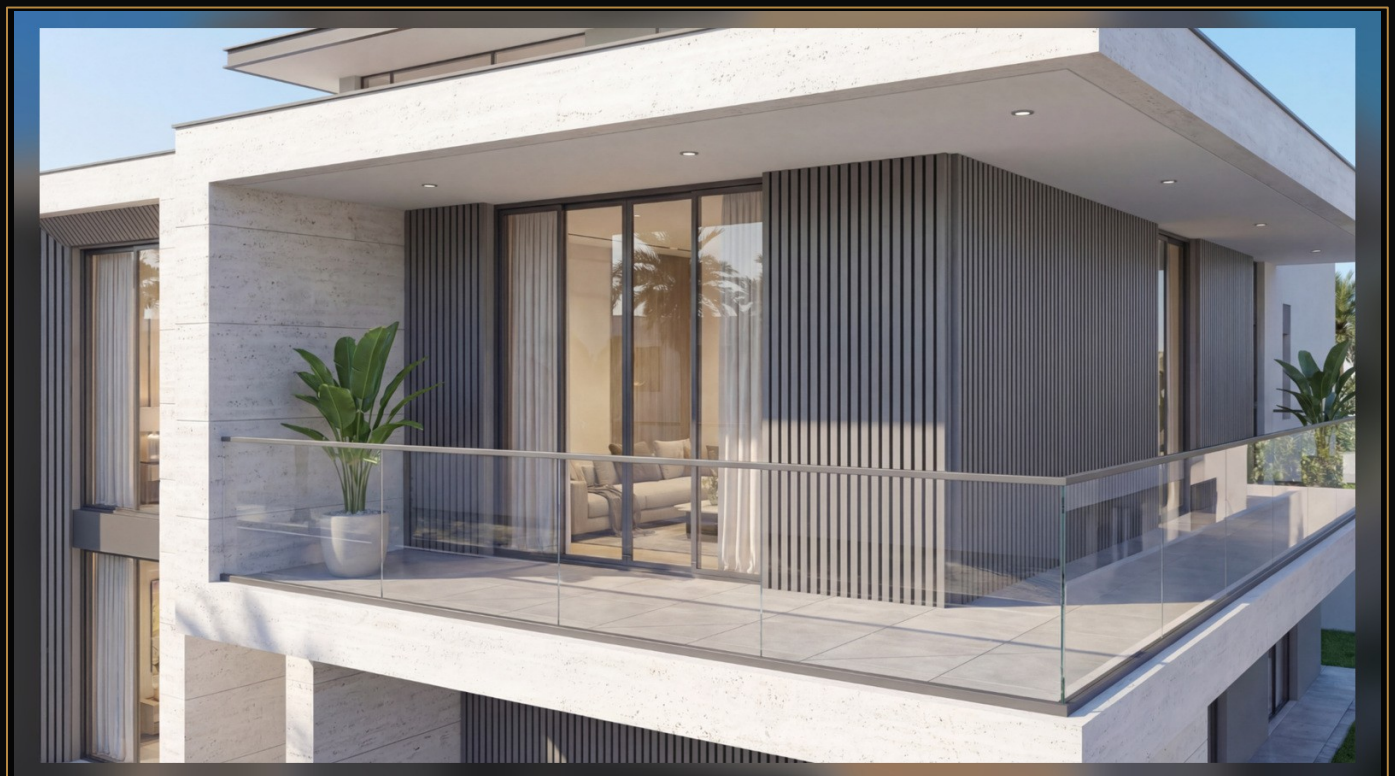
Upper terrace with glass balustrade and privacy fins
